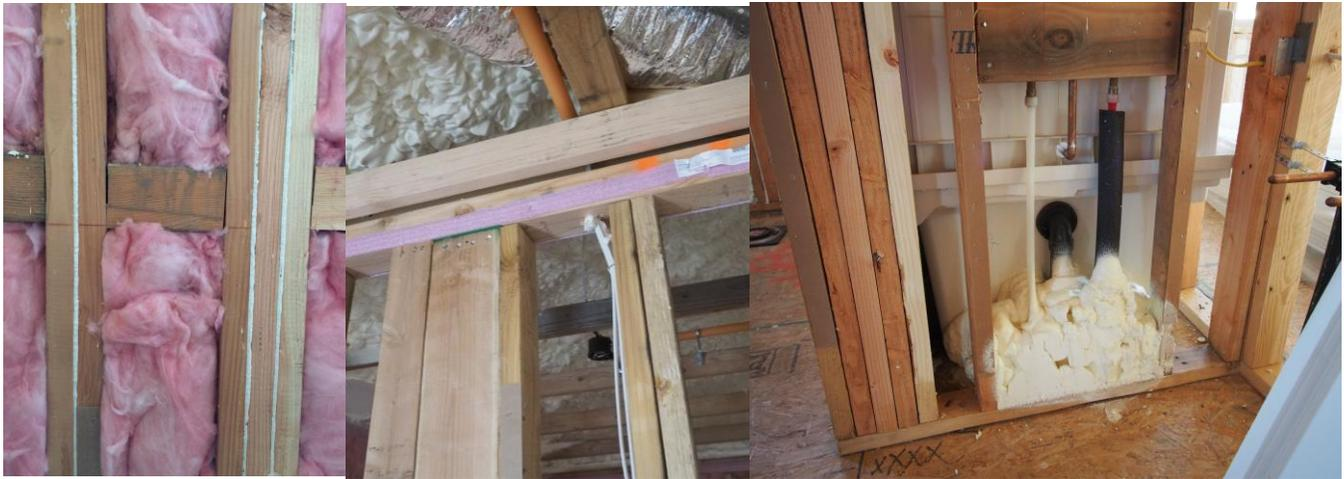
Can foam used between double studs      Foam gasket to seal drywall between house and attic      Spray foam used at plumbing penetrations
