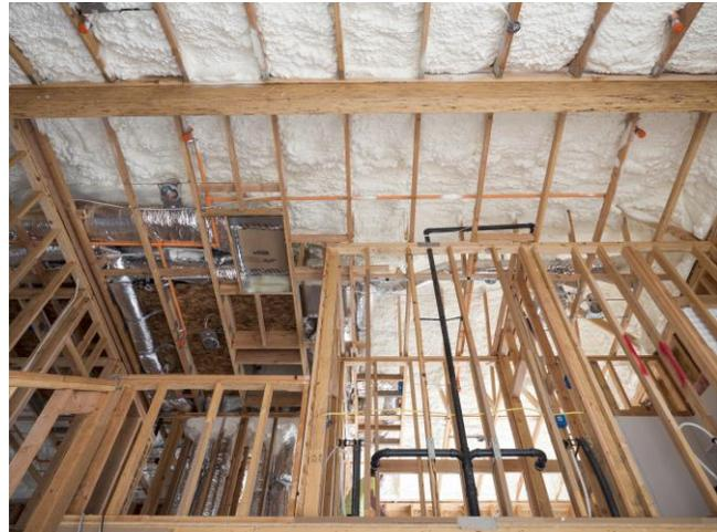
Open-cell spray foam installed below roof deck
