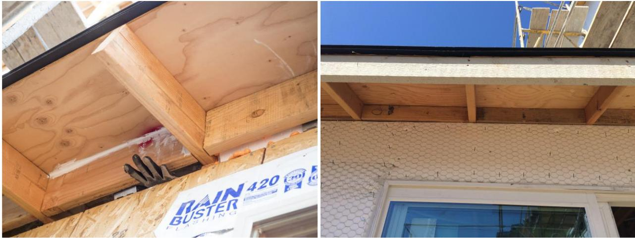
Figure 7. Gap at eaves requiring manual blocking prior to AeroBarrier (left), example of exterior ridged foam used to close the gap prior to open-cell spray foam installation (right)
