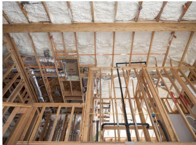
Open-cell spray foam installed below roof deck
