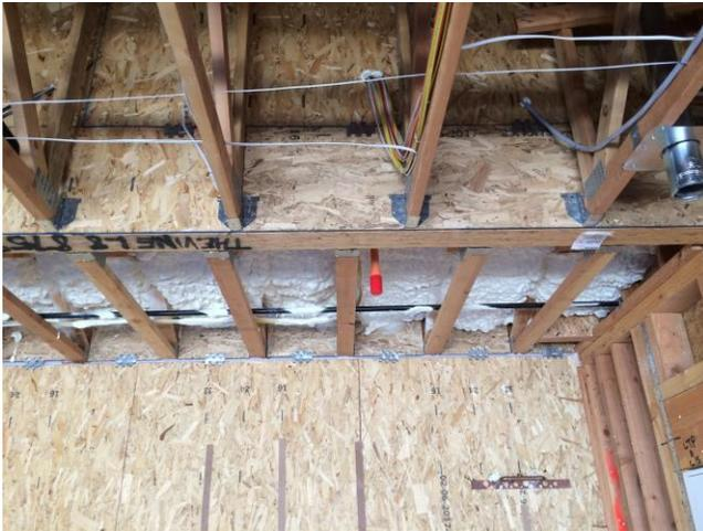
Open-cell spray foam installed at rim joist
