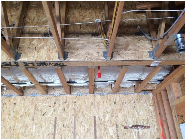
Open-cell spray foam installed at rim joist
